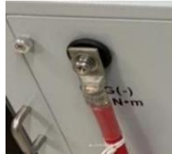
Battery Termination at Terminal
