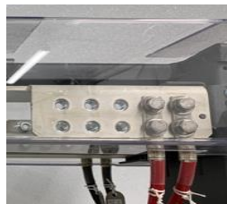
Busbar Termination Terminal
